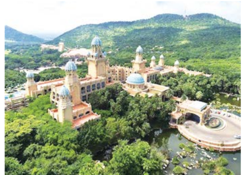
4. The Palace of the Lost City hotel is the biggest theme resort hotel in the entire world and is the largest building project undertaken in the southern hemisphere.
