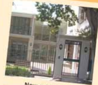
New entrance to Rosecourt / Vriende residence
